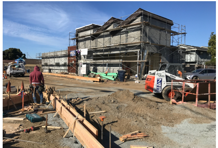
Progress on the future Mayou Family Center, 2019
